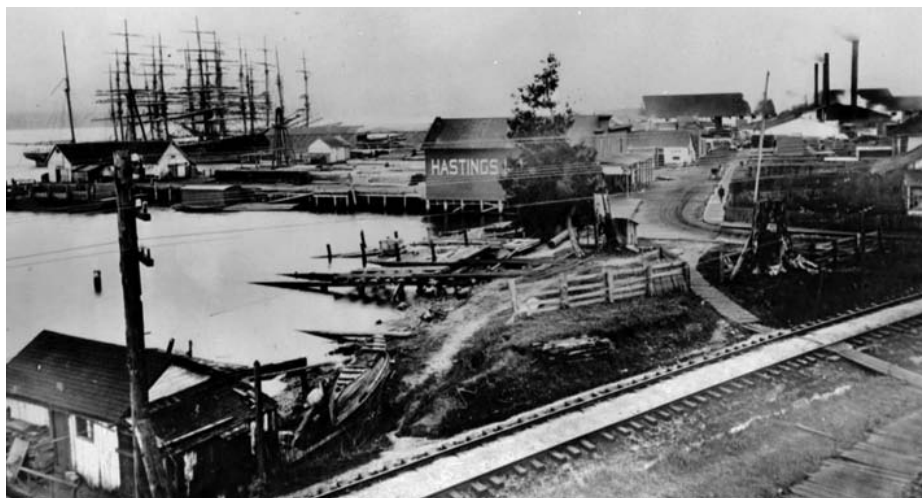
FIGURE 6–21 Hastings Mill in the 1880s. Considering raw resources, workers, and the export of products, why might a lumber mill be successful in this area?
