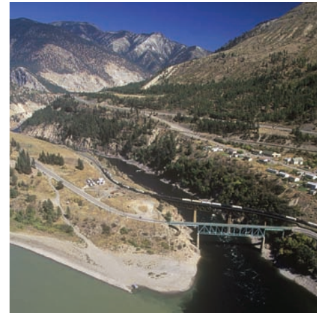
FIGURE 6–8 The Lytton Bridge was renamed the Chief Spintlum Bridge in honour of Cxpentlum.
